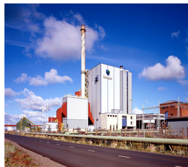
Kokkola power plant. Photo: Fortum
